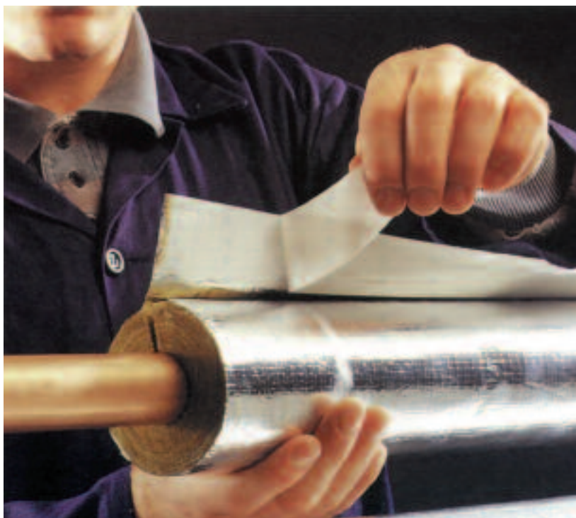
Fast installation of Rockwool Rocklap H&V Pipe Sections to copper pipes
